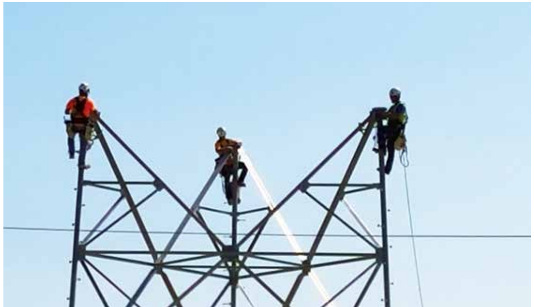
Installation of 911 Emergency System in Kentucky.
