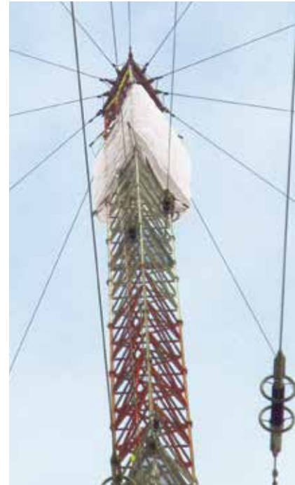
Painting of 827' tower in Italy. Photo below shows the outside view of the project while in progress.
