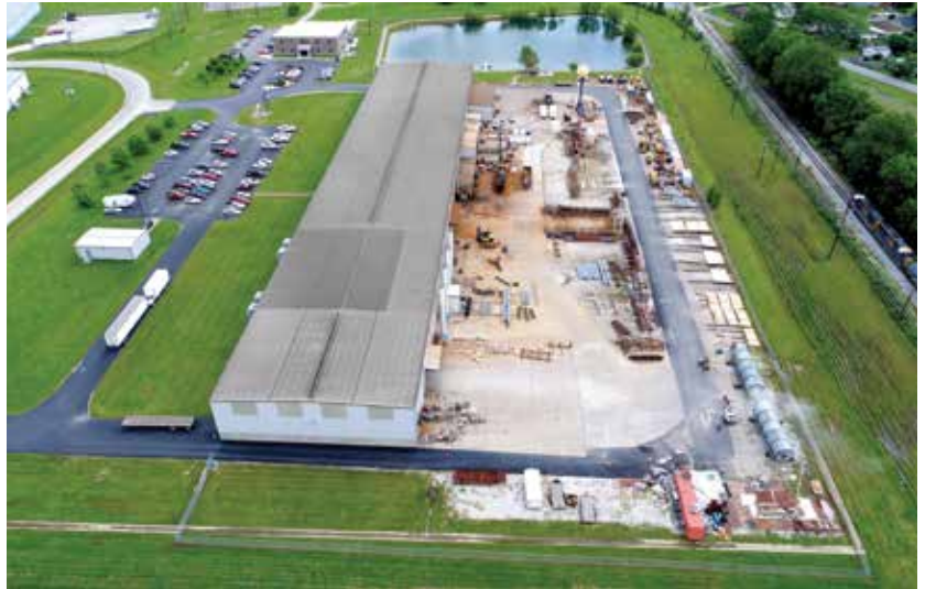
Pittsburg Tank & Tower manufacturing facility located in Henderson, Kentucky. 110,000 sq. ft. facility on 22 acres.
